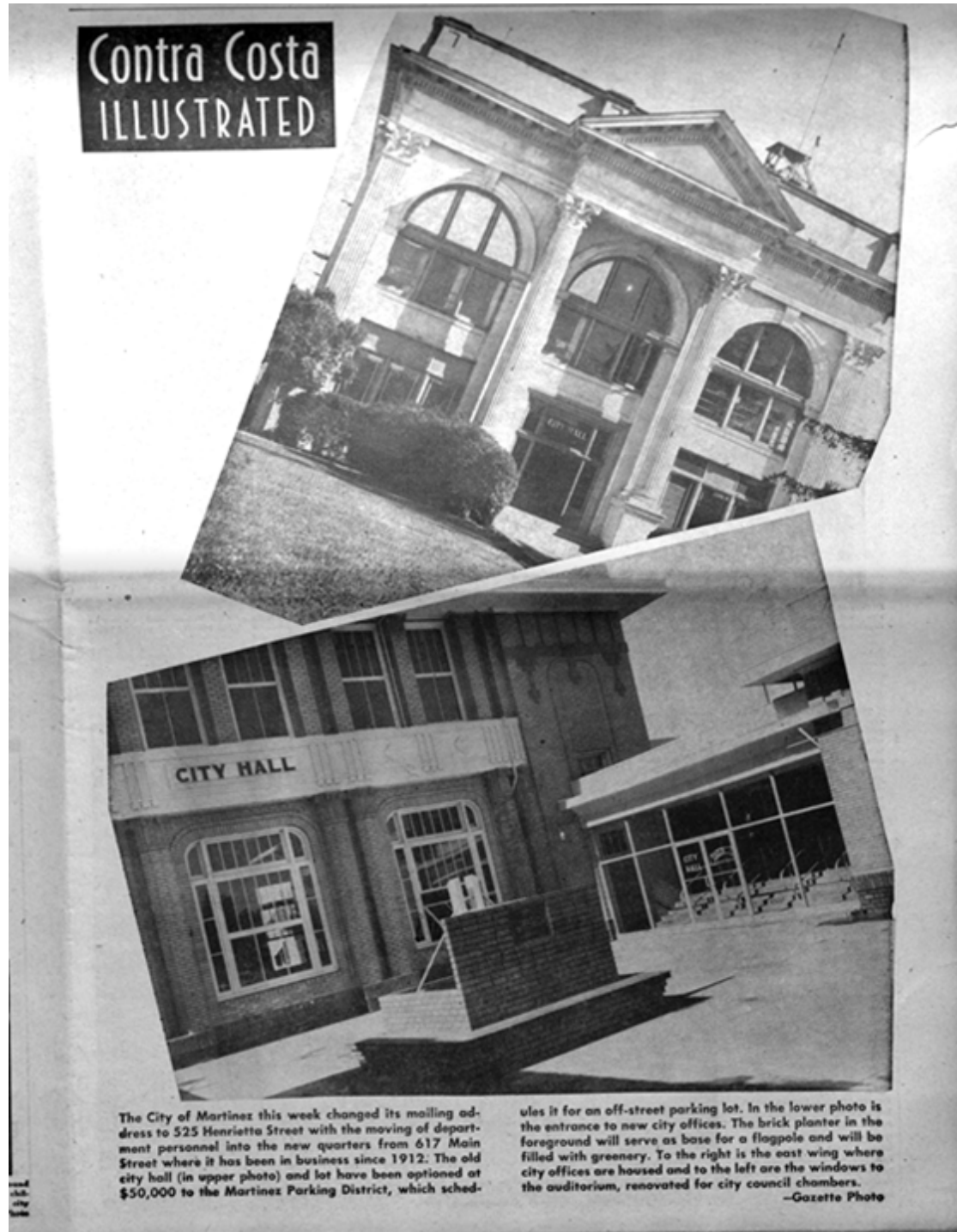
Figure 13. Central entrance arch no longer contained a door, 1956; Contra Costa Gazette Photographer, Courtesy Contra Costa Historical Society
