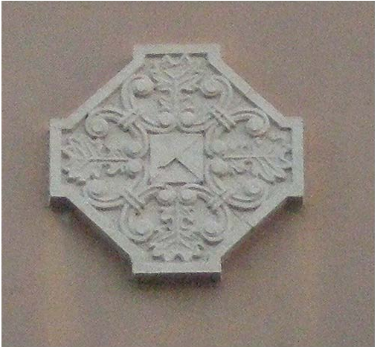
Figure 23. Sullivanesque ornamental medallion adhered to Martinez City Hall lobby exterior (main massing spandrel), 2017. Photographer: Rob Parolek, City of Martinez Park, Recreation, Marina, & Cultural Commission
